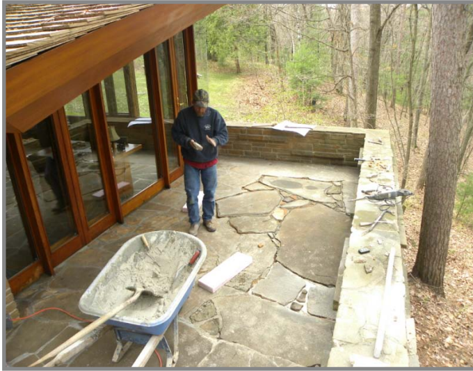
Work Week 2010 included resetting the terrace flagstones...
