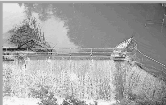
Mirror Lake dam during the flooding of June 2008.
