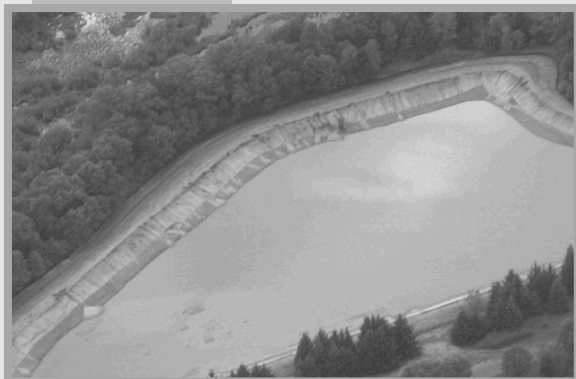
Sediment storage area.
