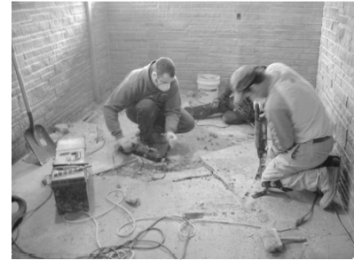
Removing the stone floors in the bedroom.
